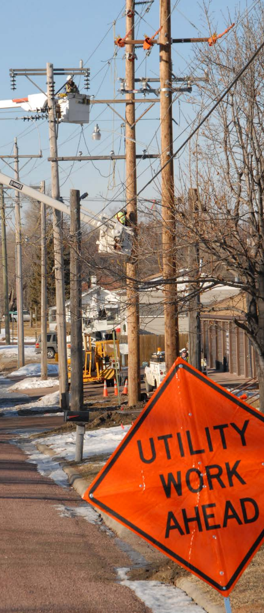
Crews work to rebuild a power line in Mitchell.
