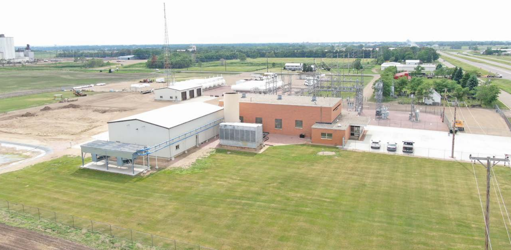
NorthWestern Energy is currently building a 60 MW generating station in Huron.
