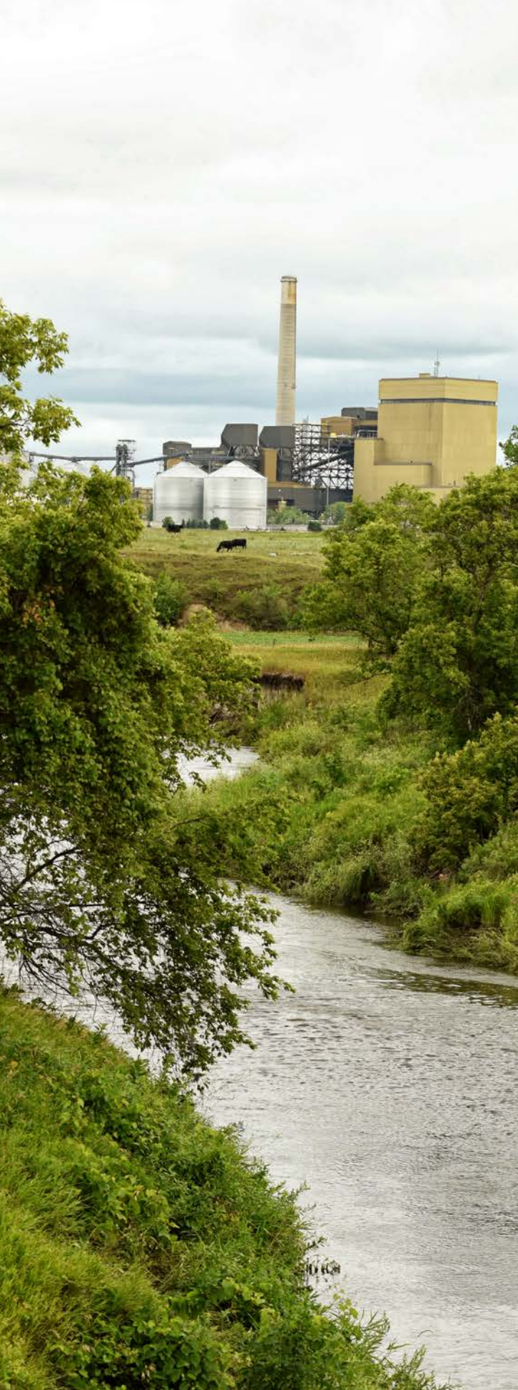
Northwestern owns 23.4% of the Big Stone Plant, coal-fired, cyclone burner, non-scrubbed base load plant.
